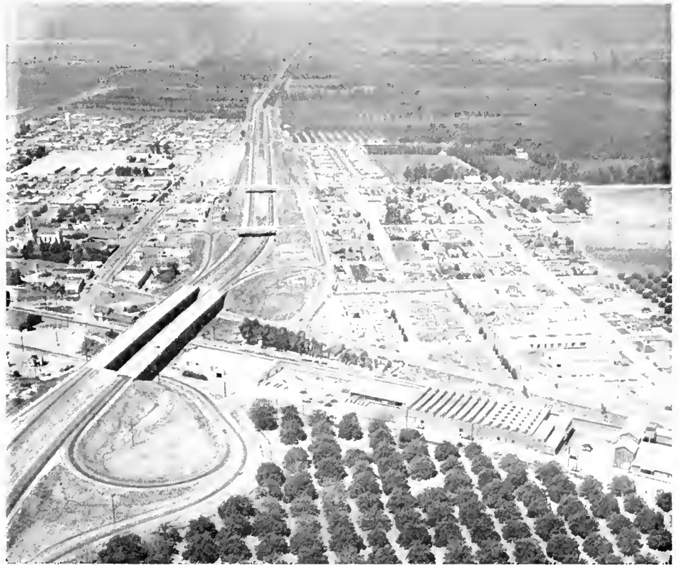
Aerial view showing freeway and old highway through center of Camarillo. Row of palm trees left of freeway indicates central portion of business district along old highway route.
